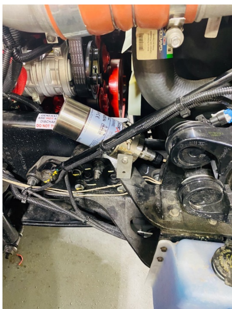
One generator on an engine compartment install.
